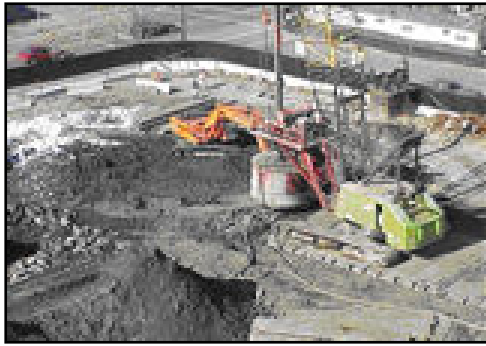
Figure 3-3. In-Situ Treatment Using Shallow Soil Mixing Method at Former MGP Site
