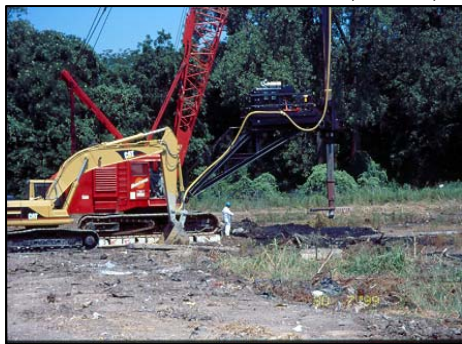
Figure 4-2. In-Situ Treatment of Sludge Pit Wastes
