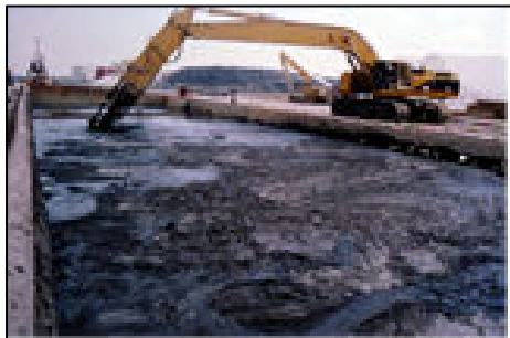
Figure 7-5. Dredged Sediment Undergoing Treatment in Barge
